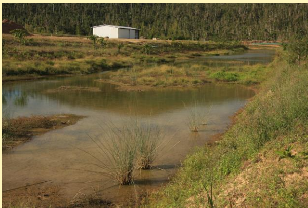
Figure 3. Silt traps are the last line of defence and prevent sediment leaving the farm
