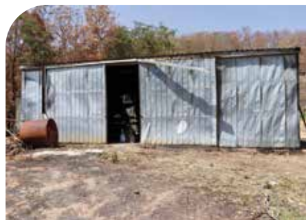
The exterior of Clinton Welsh's packing shed, destroyed by fire.
