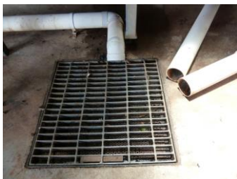
Grates in the packing shed remove banana flowers and other debris effectively from waste water.
