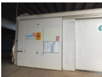
Regularly check cold room seals to make sure they are not losing air.
