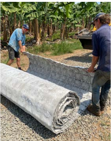
◀ Installing concrete mats at Tropicana's Kalbo farm. Picture courtesy of Gavin Eilers.
