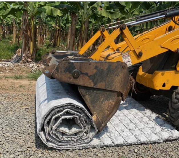
◀ Installing concrete mats at Tropicana's Kalbo farm. Picture courtesy of Gavin Eilers.
